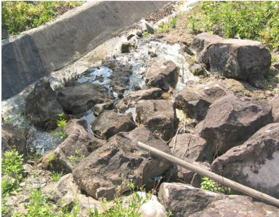
(c) On-site water leakage phenomenon 1.
