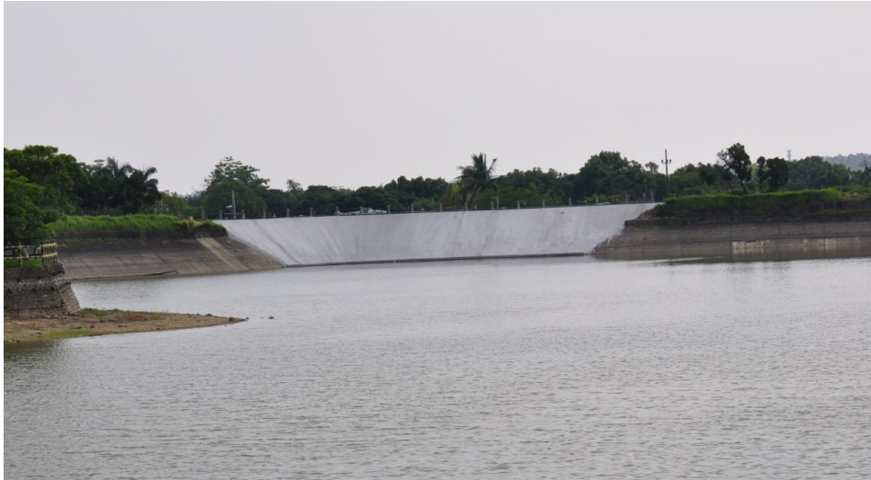
Figure 16. The turning point of the Hutoupi Earth Dam after completion of the restoration project (August 2016).
