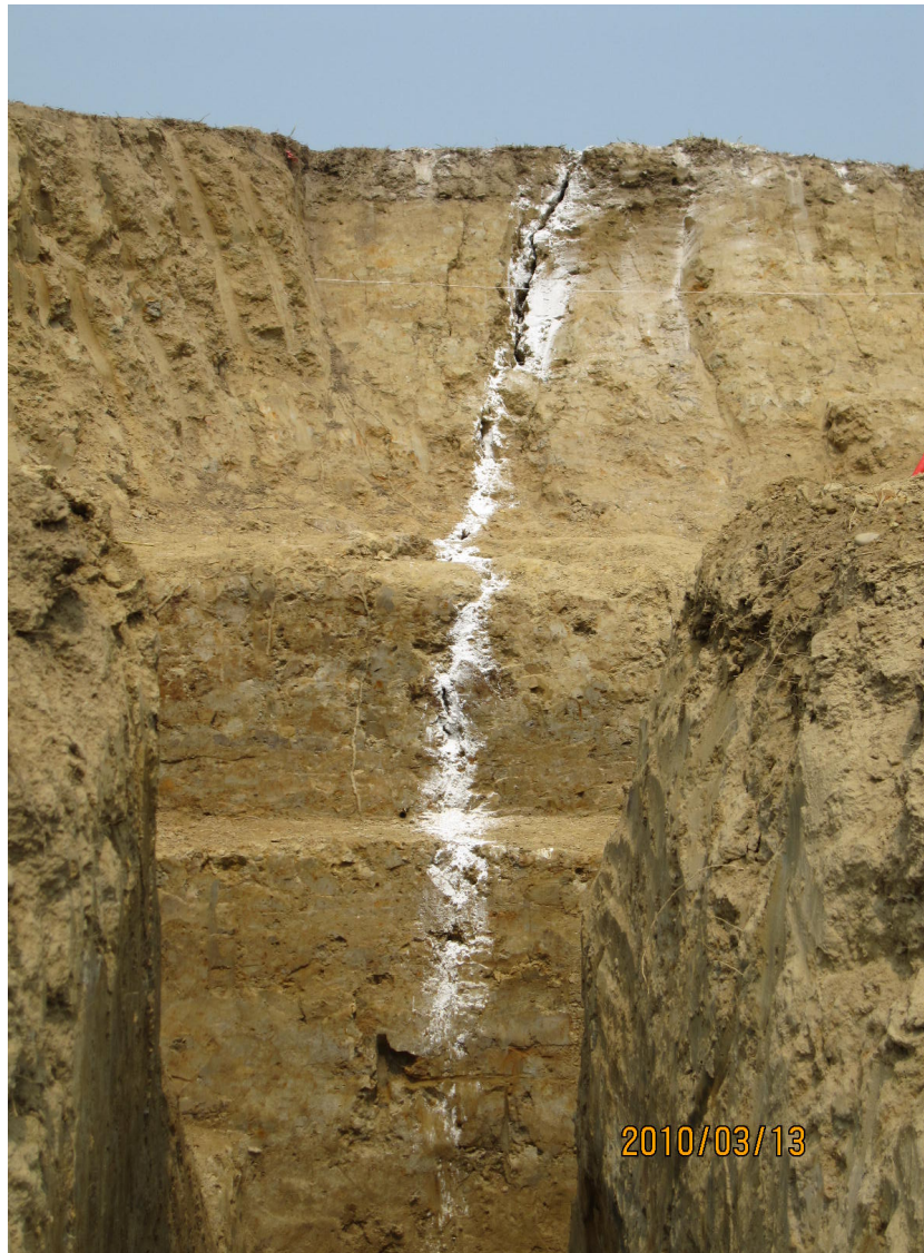
(b) The results of the investigation using in-situ excavation methods.
