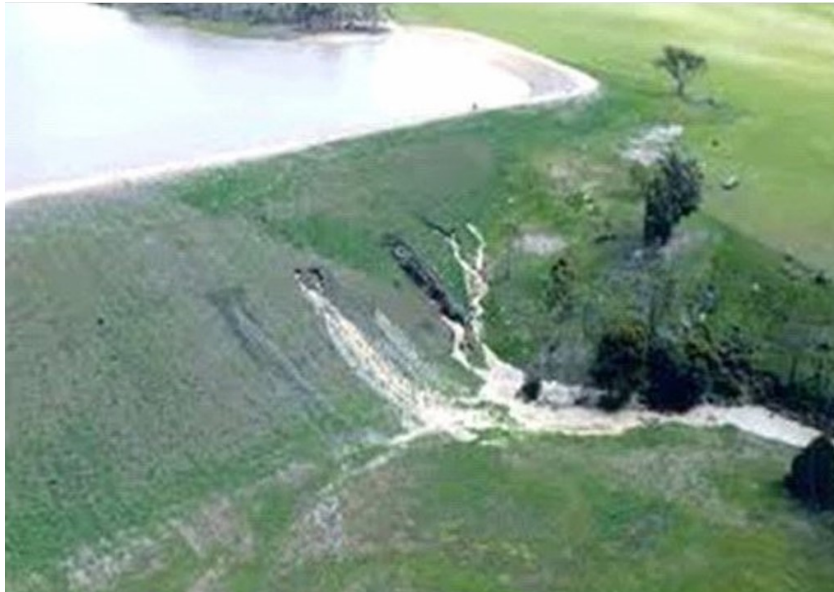
Figure 2. Example of piping failure at the turn of an earth dam (Wendy Fisher, 2021).
