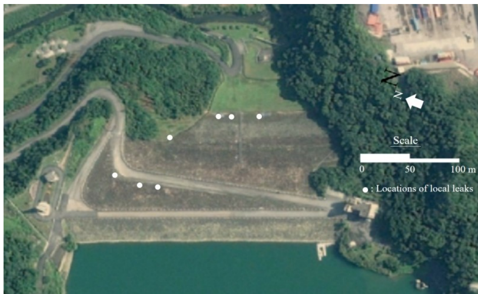
(b) The location of the leak in the earth dam (Google Earth, 2021; Data from Lin, 2009).
