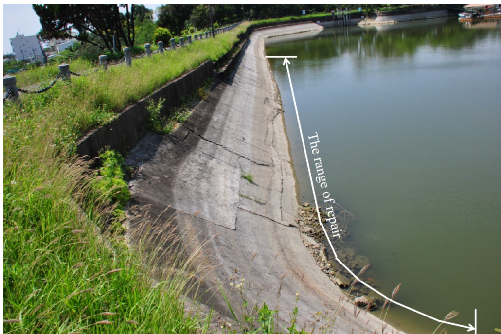
Figure 14. Longitudinal repair range for the Hutoupi Earth Dam turn.
