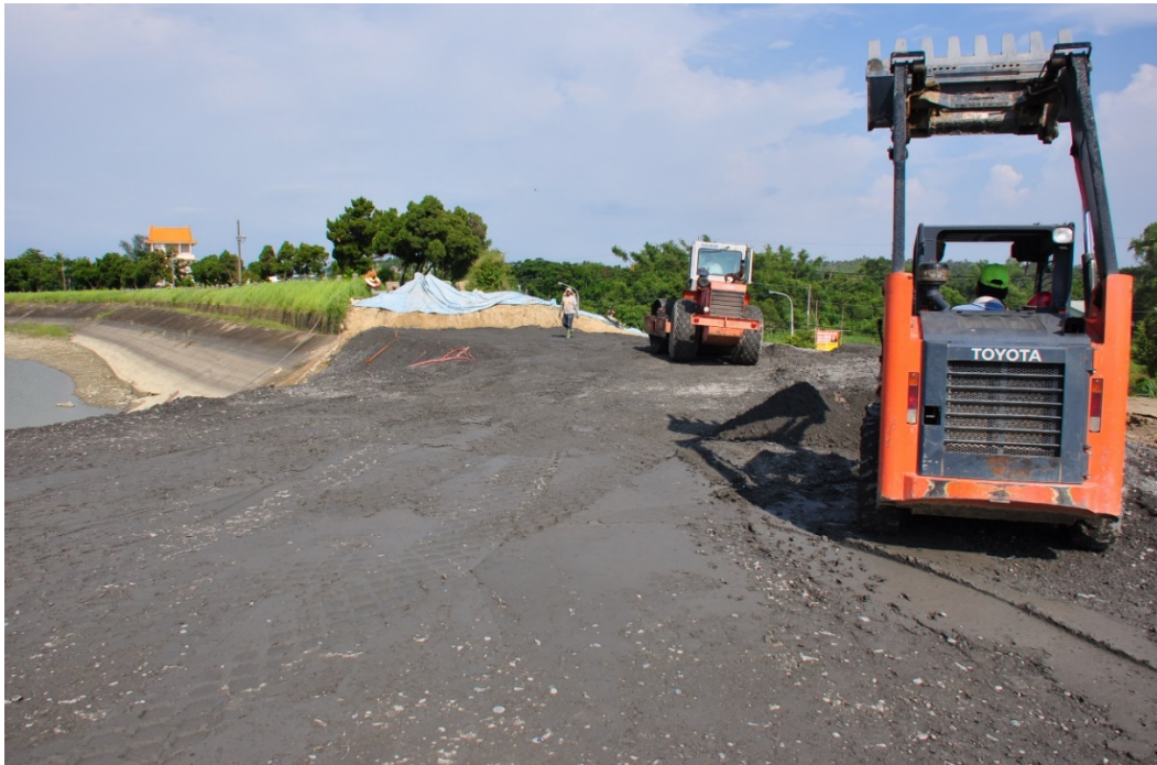
Figure 15. Rehabilitation of the turn of the Hutoupi Earth Dam after the Meinong earthquake.
