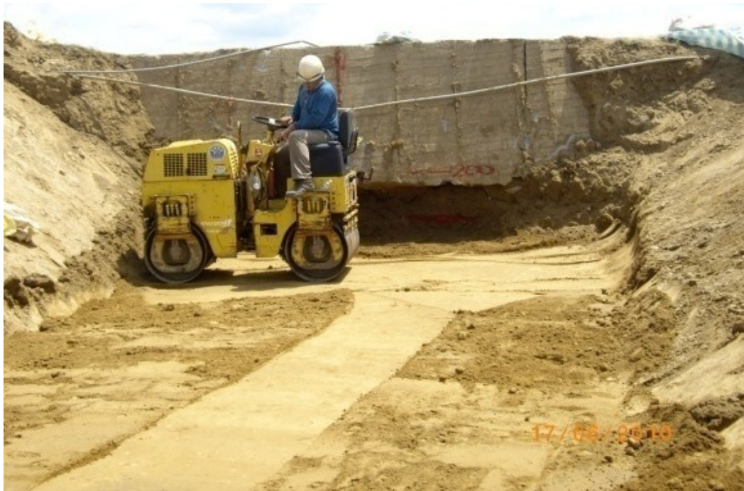
Figure 8. Layered backfilling and rolling operations for the Jiaxian Earthquake Restoration Project of the Hutoupi Earth Dam (Jianan Farmland Water Conservancy Association, 2012).
